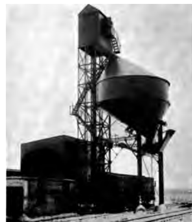
150 Ton all Steel Coaling Station
